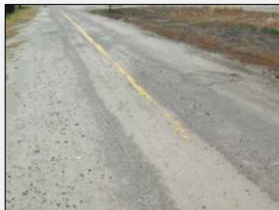
Asphalt deterioration
