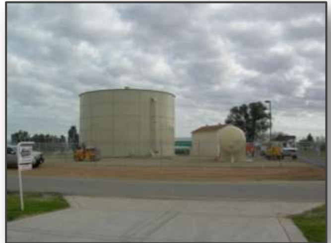
New water storage tank
