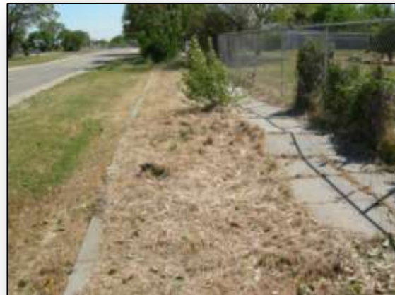
Buckling sidewalk
