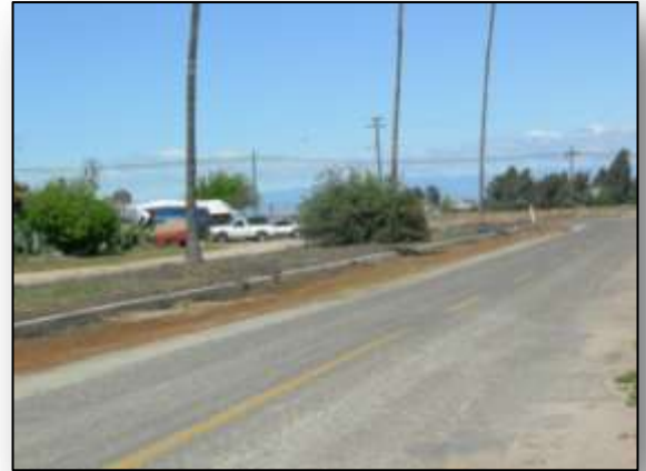
Wide median on Sinclair Drive, unmaintained
