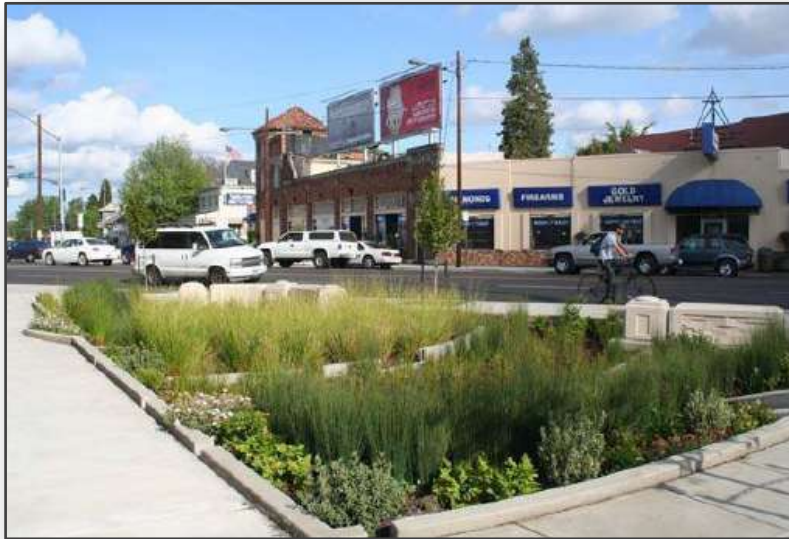
A rain garden utilized to collect stormwater in a commercial area. Source: Opticos Design, Inc.
